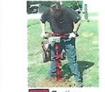
11 Continue digging with auger and extension.
